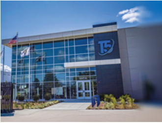
T5 Data Center - Elk Grove Illinois
